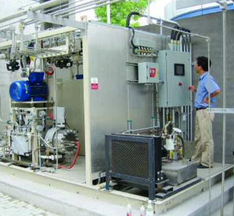
BOC/Linde used a PDC compressor in its joint venture to build 1st Shanghai hydrogen station in collaboration with Tongji University & Shell.
