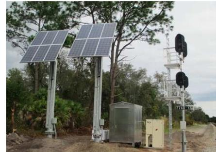
Fuel cell co-located with solar to power railroad safety signaling equipment in Florida
